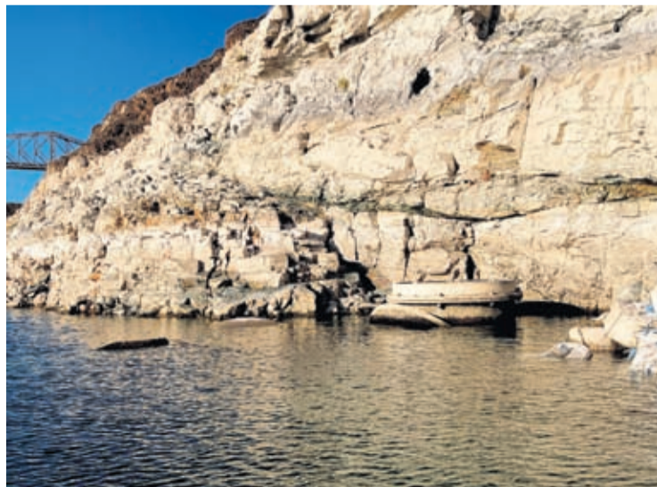
This April 25, 2022 photo provided by the Southern Nevada Water Authority shows the top of Lake Mead drinking water Intake No. 1 above the surface level of the Colorado River reservoir behind Hoover Dam.
